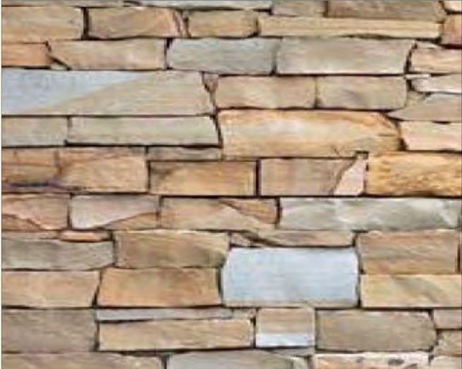
4" ANCHORED STONE VENEER OPTION 1- VARIEGATED CRAB ORCHARD IN RANDOM LINEAR ASHLAR COURSING
