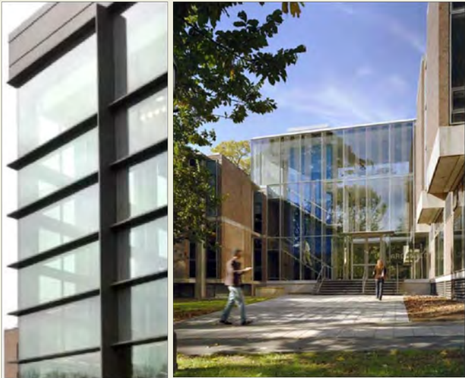
CURTAIN WALL SYSTEM-HIGH PERFORMANCE WITH NEUTRAL COLOR GLAZING AND BRONZE METALS
