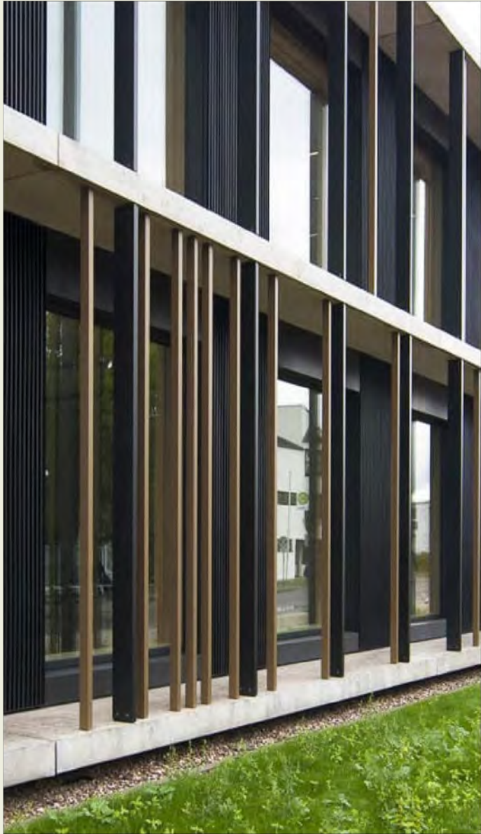
HIGH PERFORMANCE STEEL COATINGS AND METAL COLUMN CLADDING- BRONZE COLOR WITH GOLD ACCENT
