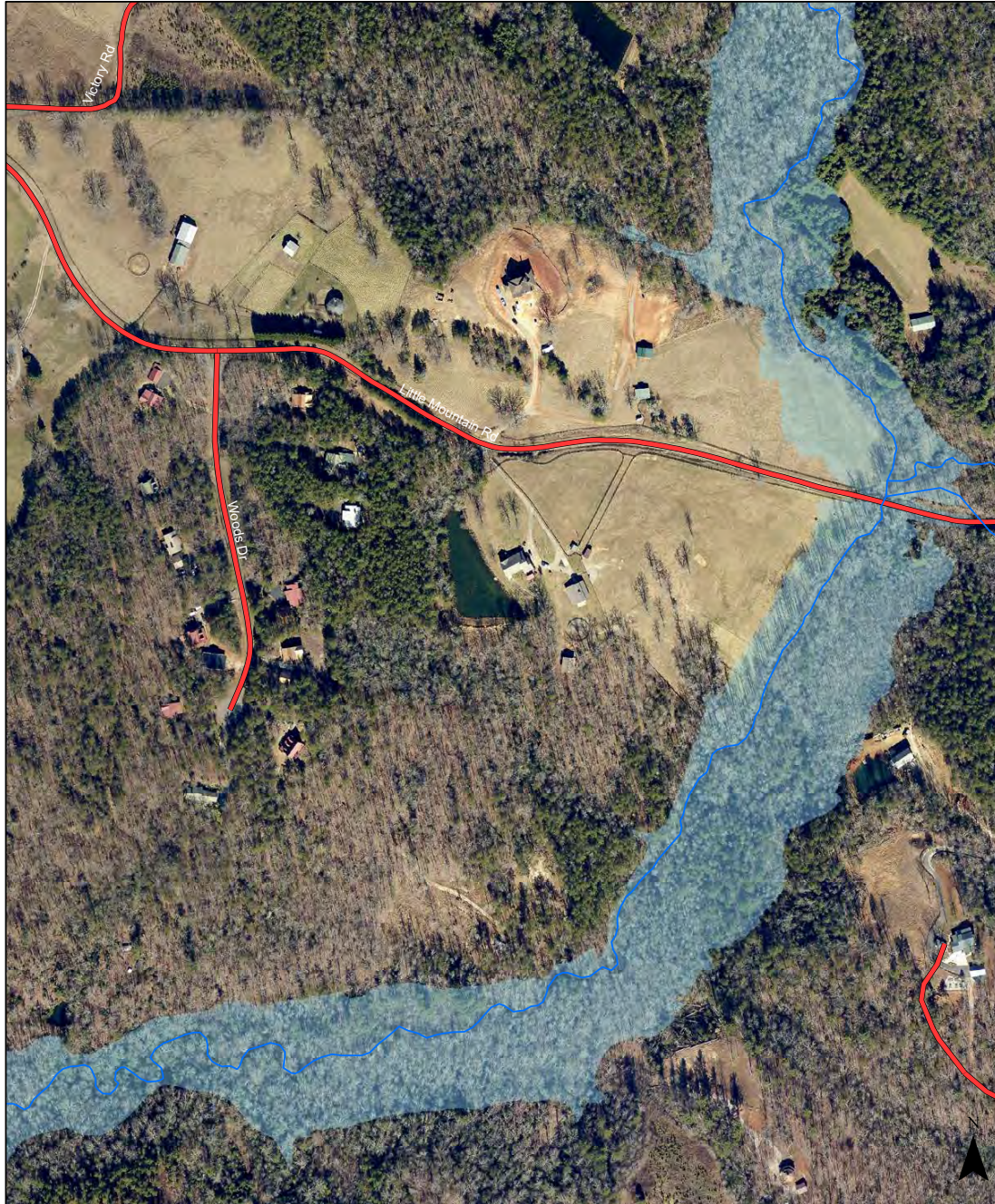
Flooding Concerns 8" over Little Mountain Road at Woods Drive
